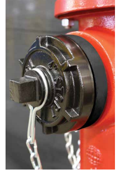
The Storz Nozzle cap can be removed with a standard hydrant wrench or Storz spanner wrench.
