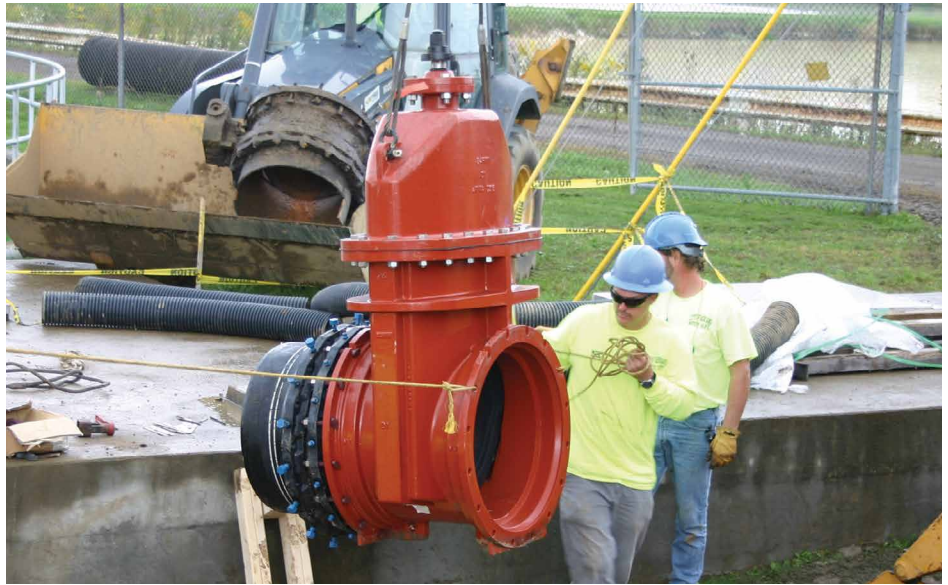
Installation of 24" resilient wedge gate valve
